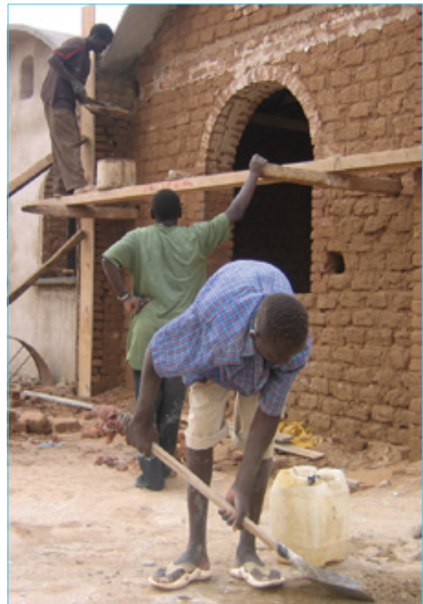
A house under construction through Sawa Sawa's credit for housing scheme
